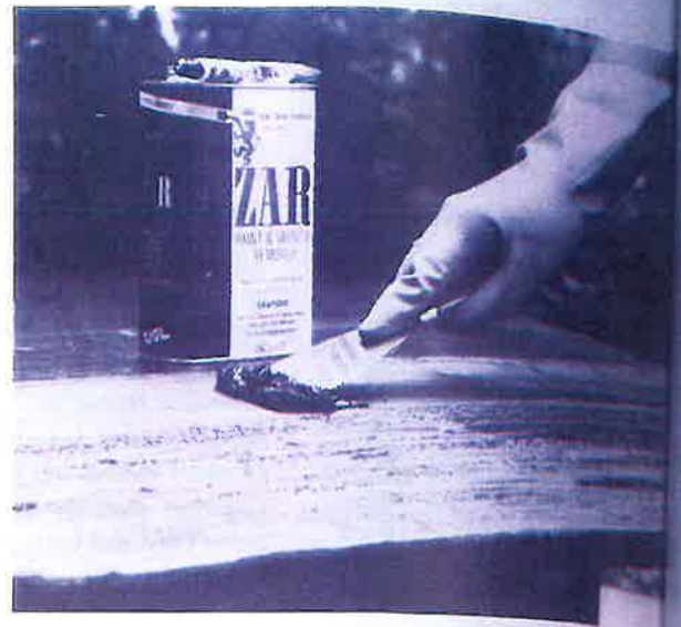
64-3(b). Using a putty knife to remove the old finish.
