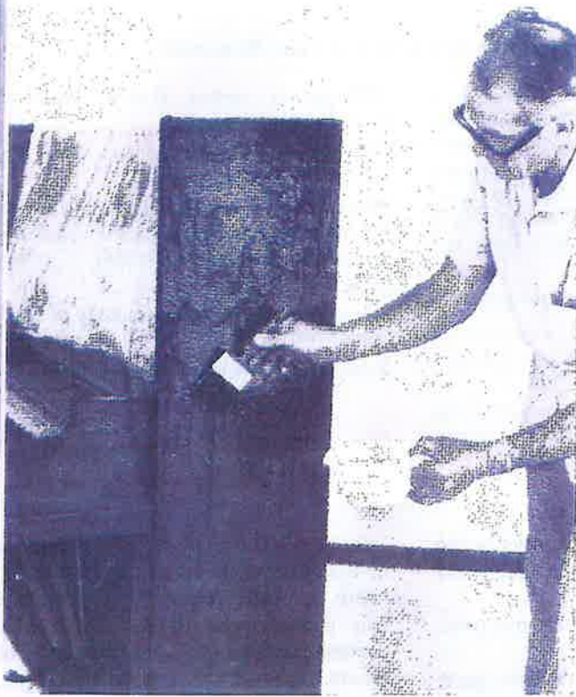
64-3(a). Apply remover as heavily as possible.
