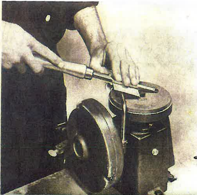
24-19(b). A fine wheel can also be used for honing.
